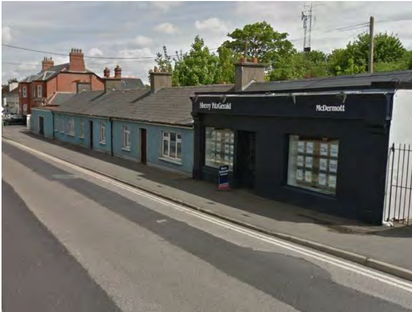
Plate 9: View of the cottages (now boarded up) from Station Road, facing northeast.
